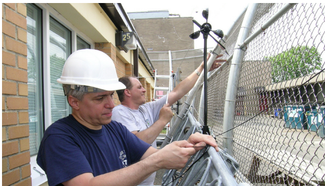
Bob Famiglio and Ray Jones prep tower for new HF vertical.
