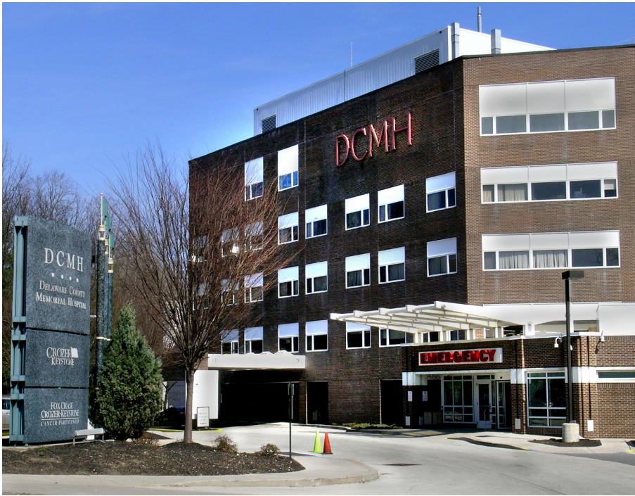
DELCO D-STAR EAST repeater system is located at DCMH in Drexel Hill, PA
